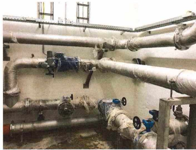
Neue Hydraulik HB Schutterlindenberg
